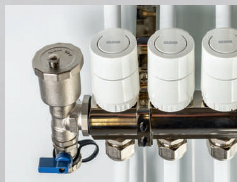
The room thermostat also controls valve drives (230 volt), which are mounted in the heating manifold.
